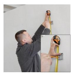
1. Measure and mark places for the installation of brackets.
